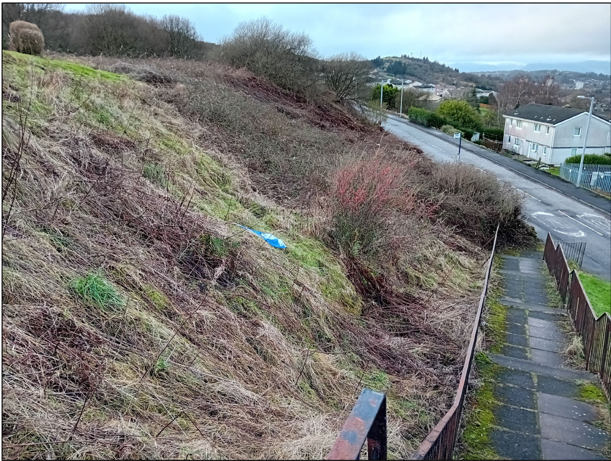
View from easternmost point of site, facing west across site.
